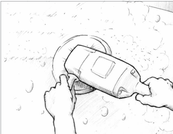
Figure 2-2 Use an electric polisher with an 8" foam sanding pad to open blister cavities or remove gelcoat.
