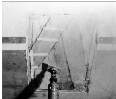
Figure 5-18 Bond the second layer in the opposite diagonal to the first layer.
