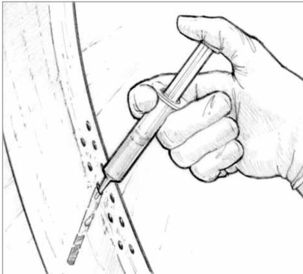
Figure 3-4 Inject resin/hardener mixture into holes until the damaged wood absorbs all it can.
