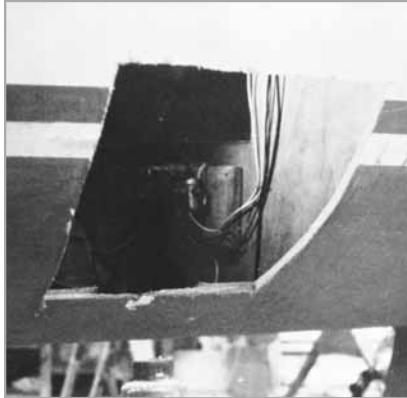
Figure 5-15 Remove the damaged section.
